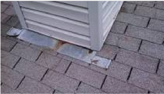
2/2/2017 photo of Deteriorated Strip Flashings
