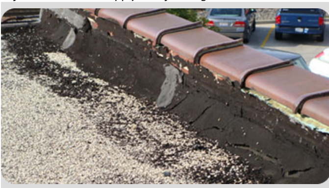
2/2/2017 photo of Deteriorated Base Flashings
