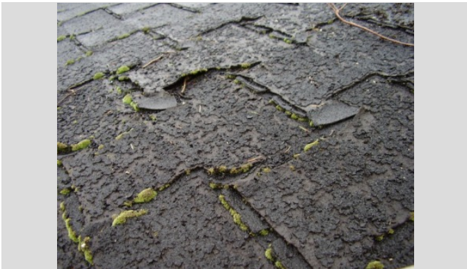
2/2/2017 photo of Blistering (no rupture)
